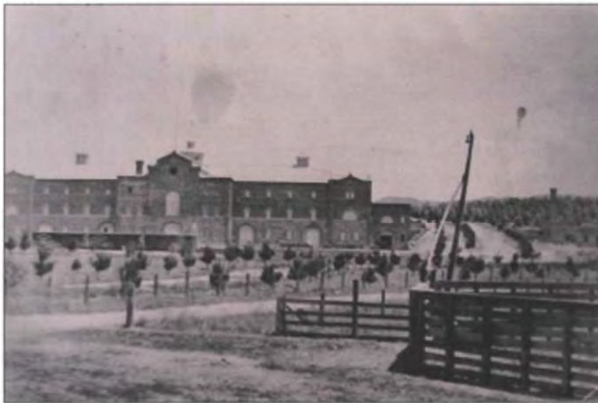
Photo 5. Gallegos Winery and grounds (Von Buskuh (?) pre-1906).
