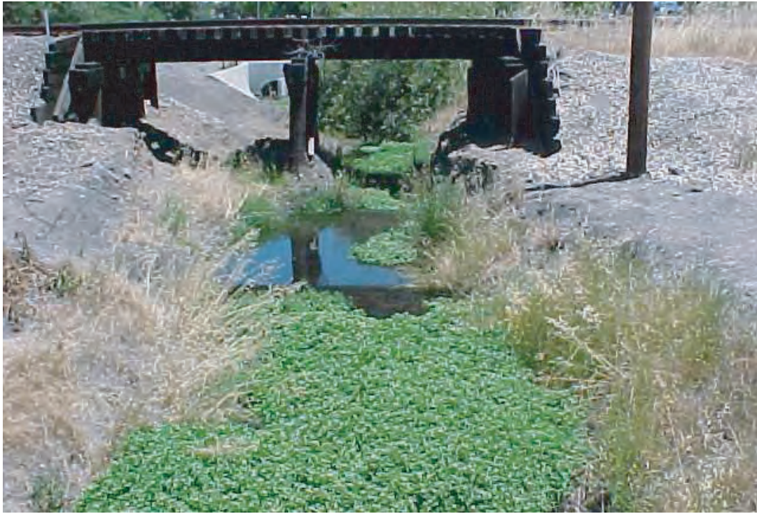
Flood control channel north of Paseo Padre Parkway
